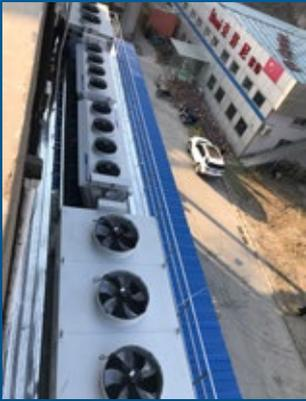
▲ At the top and bottom of the image: Gntner Flat VARIO flatbed gas coolers of type GGHV, which perform the initial stage of CO<sub>2</sub> cooling and heat recovery by cooling the hot gas from between 121 °C and 103 °C/ 249.8 to 217.4 °F down to 41 °C/ 105.8 °F with this design.
