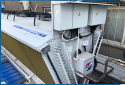
▲ A Gntner V-SHAPE compact gas cooler of type GGDC is sprayed when the outside temperature rises above 20 °C/68 °F, thus reliably cooling the hot CO<sub>2</sub> gas from 41 °C/105.8 °F to 34 °C/93.2 °F with this design.
